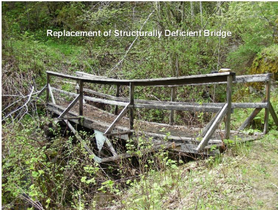
Figure 5 Typical bridge on recreation trails at Dworshak.
